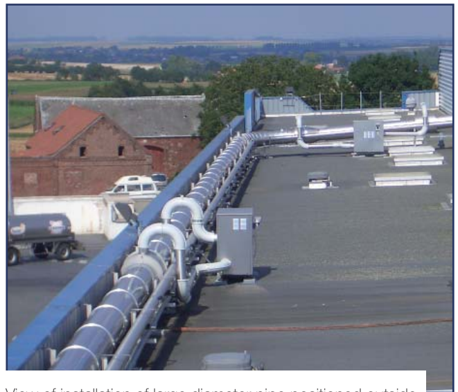
View of installation of large diameter pipe positioned outside
