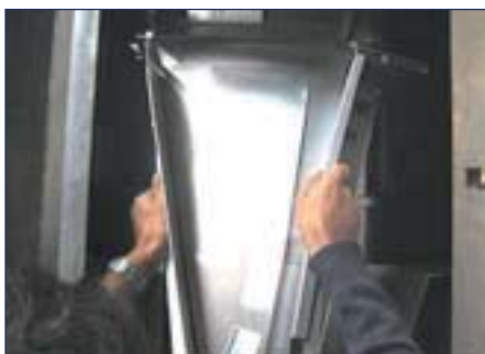
phase number 6 The funnel is installed
